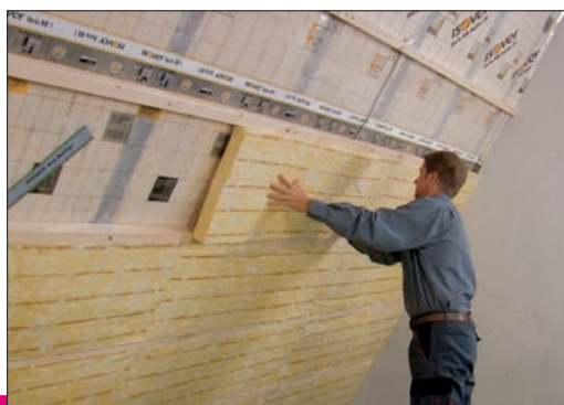
Example of product application Isover MULTIMAX 30
